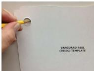
Once the location for the Control Box, Reelcraft Reel and Cleaning Solution Tank have been decided, use the appropriate mounting templates to locate and drill the required holes into the mounting surface. Use the appropriate stainless steel bolts to fasten each component to its mounting surface. Make sure to use both the flat and lock washers provided and to securely tighten.
