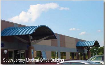
Building on the strength achieved with .050 aluminum curved ZIP-RIB roof panels, it is possible to either greatly reduce or eliminate the need for curved rafters and/or purlins in certain canopy applications. Free-Span canopies can be safely designed to spans of 16 feet without intermediate purlins. Available in 12" or 16" wide panels. Contact M&E for your specific design requirements.
