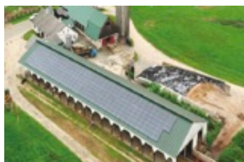
55 kW Roof Mounted Solar
