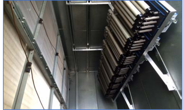
AtmosAir in RTU Discharge Plenum
