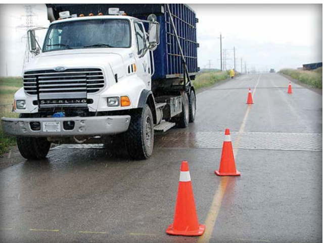
Figure 2. The pavement test track at the Waterloo Regional Waste Facility enabled four crosswalks to be installed and to rapidly receive loads from trucks.
