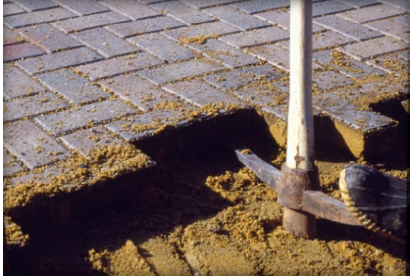
Figure 6. Prying out the remaining pavers
