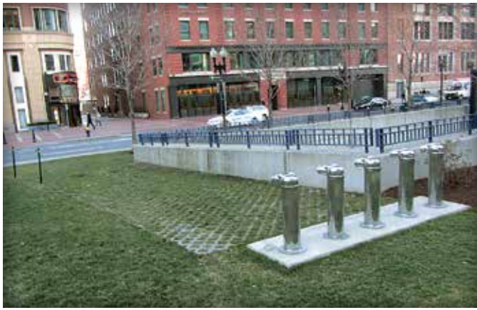
Figure 7. Emergency access lane for fire trucks
