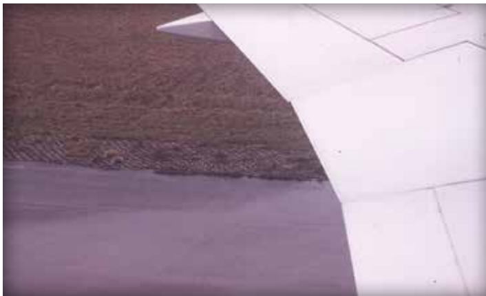
Figure 11. Airfield taxiway shoulder
