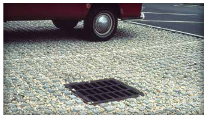
Figure 16. Concrete grids with aggregate in the openings
