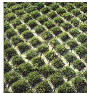
Figure 1. Grids first used in Germany in 1961 for overflow parking were building blocks placed in the ground. They emerged from the need to cool cities and decrease stormwater runoff.
