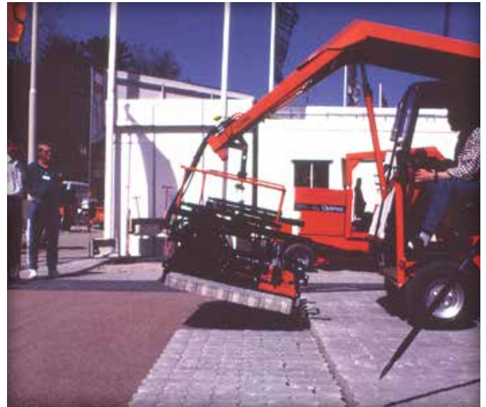
Figure 22. After the layers are separated they can be grabbed by the machine clamp.
