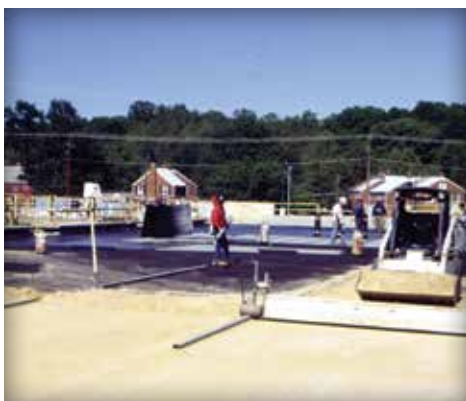
Figure 18. A mechanical screed used to level bedding sand on a roof parking deck project.
