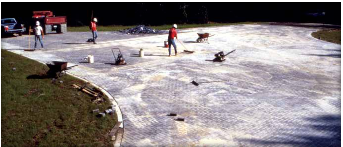
Figure 12. Excess sand swept from the finished surface will make the pavement ready for traffic.
