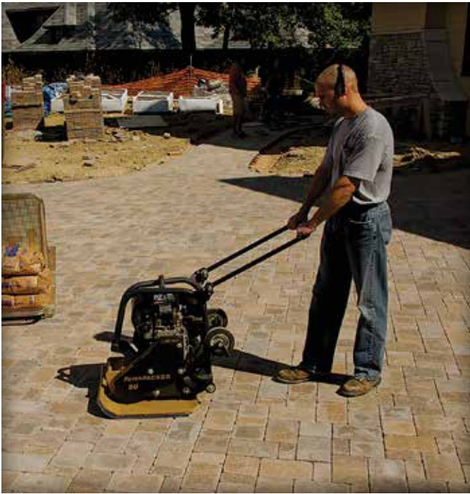
Figure 9. Compacting the pavers and bedding sand.
