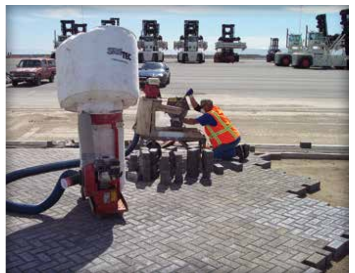
Figure 8. Saw cutting pavers.
