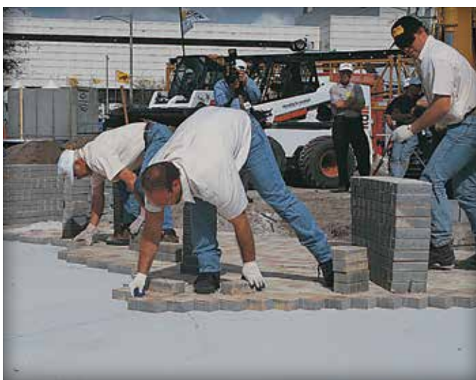
Figure 7. Placing the concrete pavers.
