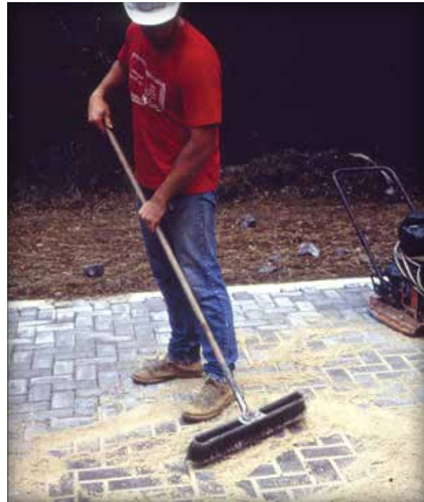
Figure 10. Spreading and sweeping joint sand.
