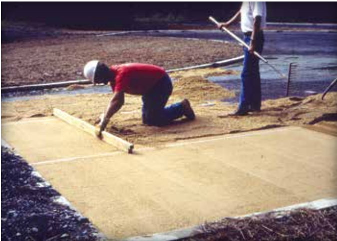
Figure 6a & 6b. Screeding the bedding sand.
