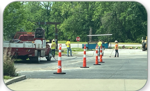
Kelpe Contracting in Labadie saw cutting a parking lot to bore in a sewer tie in.
