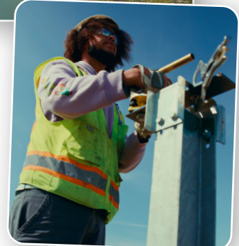
Laborers working on the Delta Bob Cat solar array.
