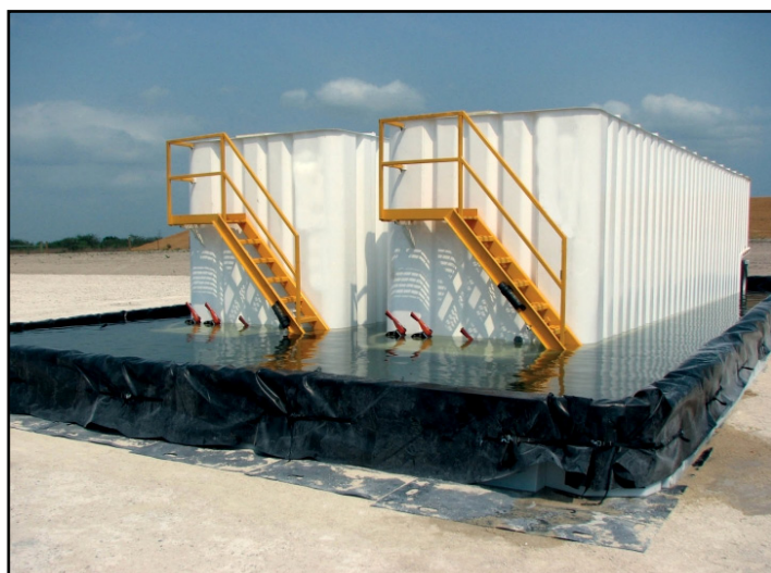
← Above ground secondary containment systems for frack tanks are used to protect against spills during hydraulic fracturing (also called “hydrofracking” or just “fracking”).
