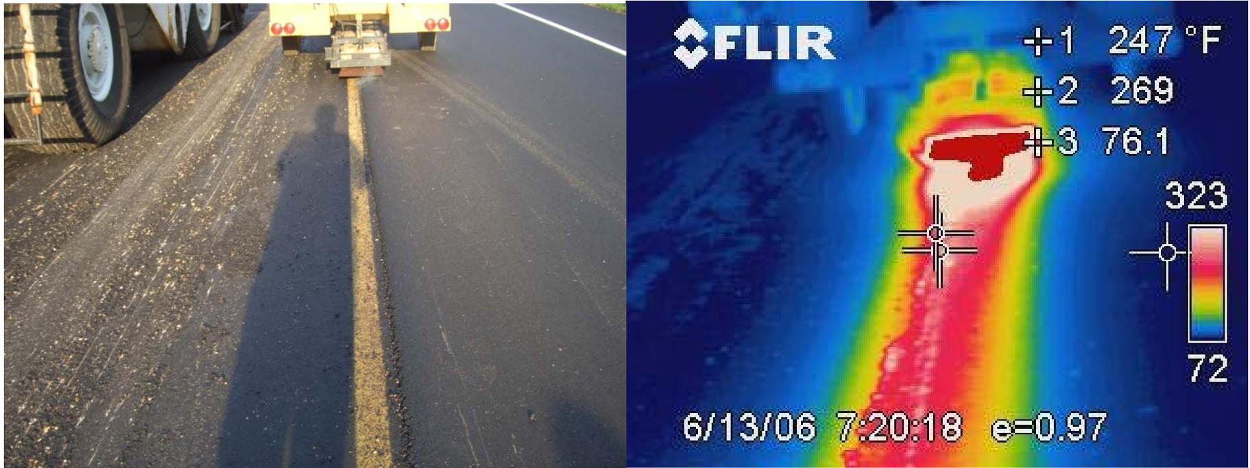
The only “smoke” is steam being driven off the surface, no evidence of blue smoke or light ends of the bitumen were noted.
