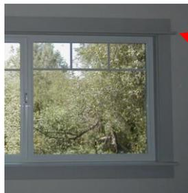
**Interior Finish Trim:** Jamb-encased installations for both interior & exterior trim details make a greatly improved appearance.
