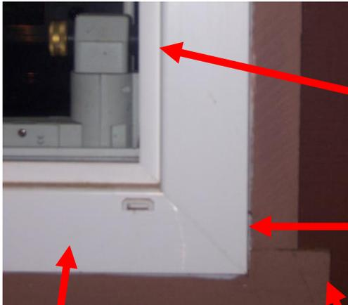
**1. Window Size:** Window height & width is reduced by +/-2 inches. Retrofit window size is reduced because the new retrofit window is mounted inside the old existing window frame.
