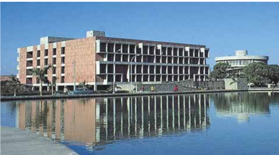
Photo 28. The Panjab University Library (left) and the Student Center (right) reflect unique, bold architectural styles.
