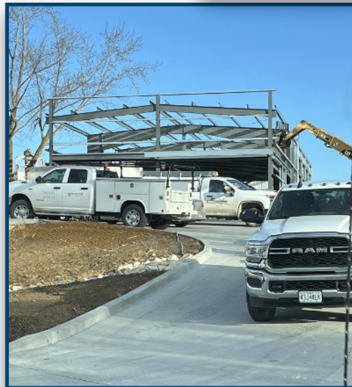
Versules Construction building an addition to Fatima School in Westphalia, MO.
