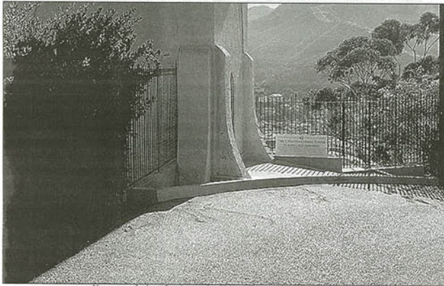
New wrought-iron fencing at the Chimes Tower. Photo by Gerry Bravo
